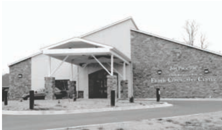
(TOP) UKB Jim Proctor Elder Community Center, Tahlequah. PHOTO WIKIMEDIA COMMONS
