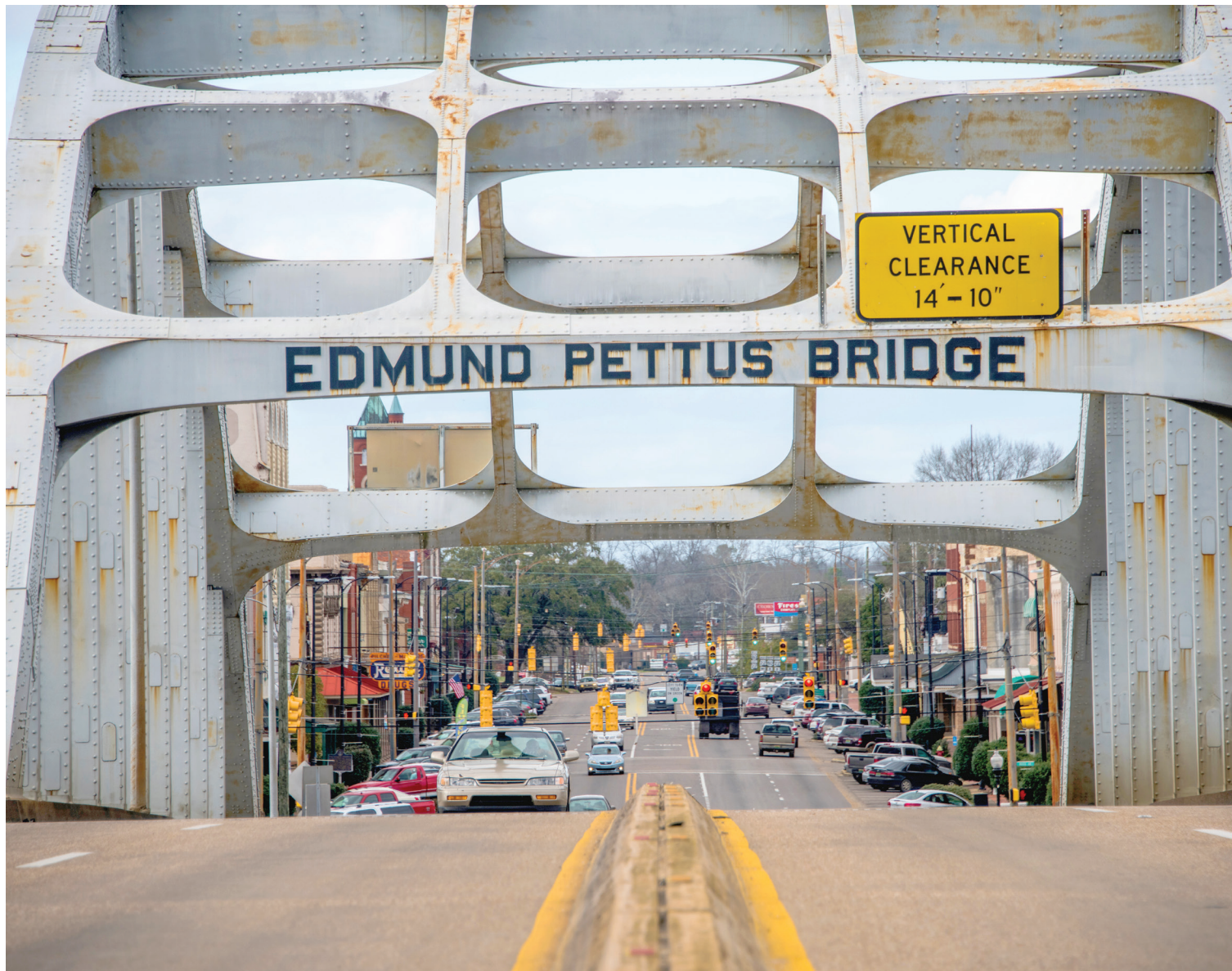
The Edmund Pettus Bridge was the site of the conflict of Bloody Sunday on March 7, 1965, when police attacked Civil Rights Movement demonstrators with horses, billy clubs, and tear gas as they were attempting to march to the state capital, Montgomery. The marchers crossed the bridge again on March 21 and walked to the Capitol building.
