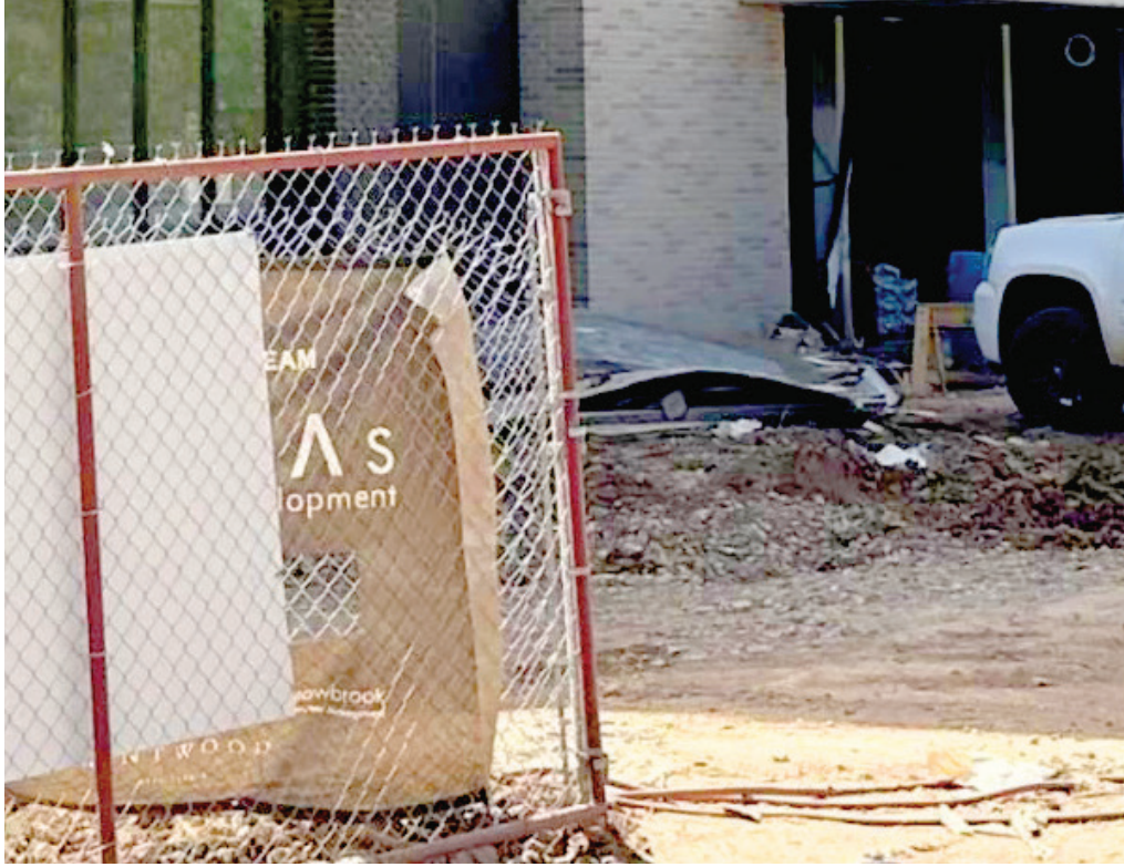
CONSTRUCTION WORKERS on basket cranes work to build a new multiplex housing unit on Northwest Expressway near Pennsylvania Ave. in Oklahoma City on April 23, 2024. PHOTO HEATHER WARLICK/OKLAHOMA WATCH
