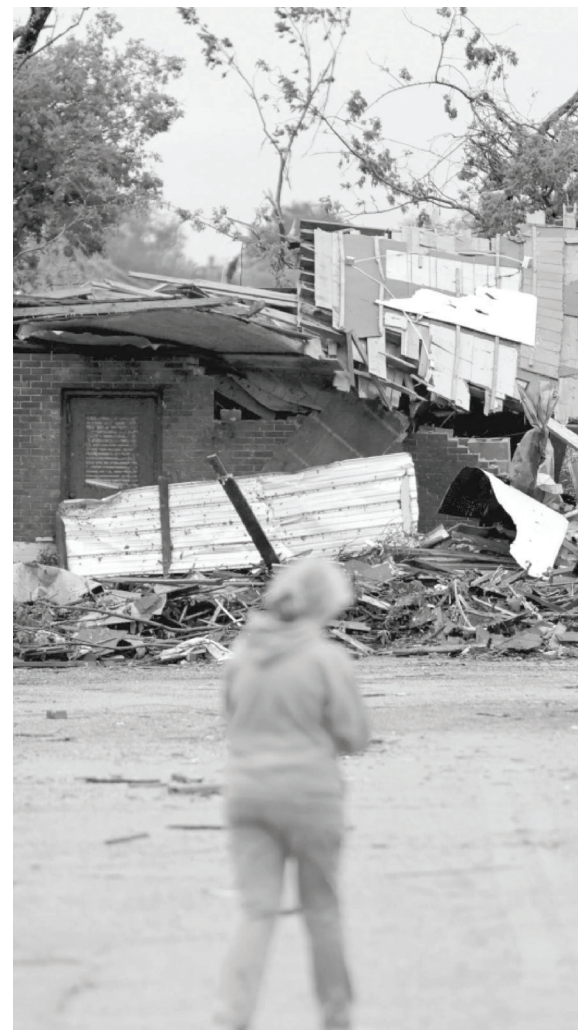
PEOPLE LOOK AT TORNADO DAMAGE IN SULPHUR, OKLA., Sunday, April 28, 2024, after severe storms hit the area the night before. PHOTO BRYAN TERRY/THE OKLAHOMAN VIA AP
